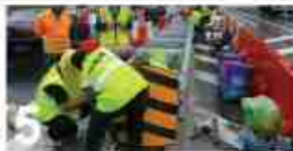
5 Attach three way slider panels, starting from the rear, using slider bolts and plates
