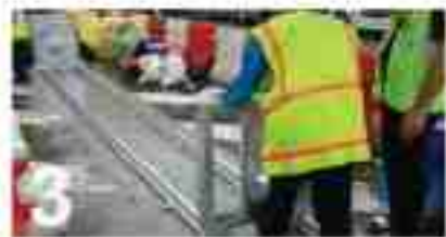
3 Slide middle supports onto rails
