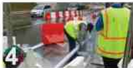
4 Slide LAF through middle supports and connect to backstop
